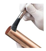
If the complete ring of solder does not appear on heating, apply additional flux to the mouth of the socket and end feed the joint with our N165 (Copper coloured) or N166 (Brass coloured) cadmium-free silver brazing alloy, or an equivalent to the compositional requirements of BS EN 1044 AG103 (formerly BS 1845 AG14).
