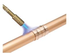
**3.** Allow the joint to cool without disturbance. Clean the joint generally, wiping off any external flux residues. This will prevent unsightly stains or (in extreme cases) corrosion of pipework. Flush out the pipework.
